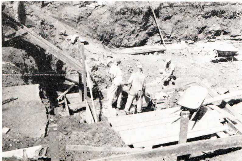
Workmen are seen pouring concrete footings for the new Dining Hall and Student Center adjoining Memorial Auditorium. Completion of the building is expected in January.
