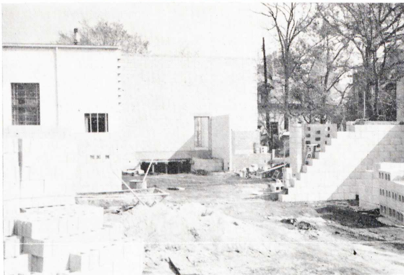
The completed walls and basement to the extension of the auditorium can be seen at the rear of the present auditorium. Materials for the dining room walls can be seen to the left and right in the picture.
