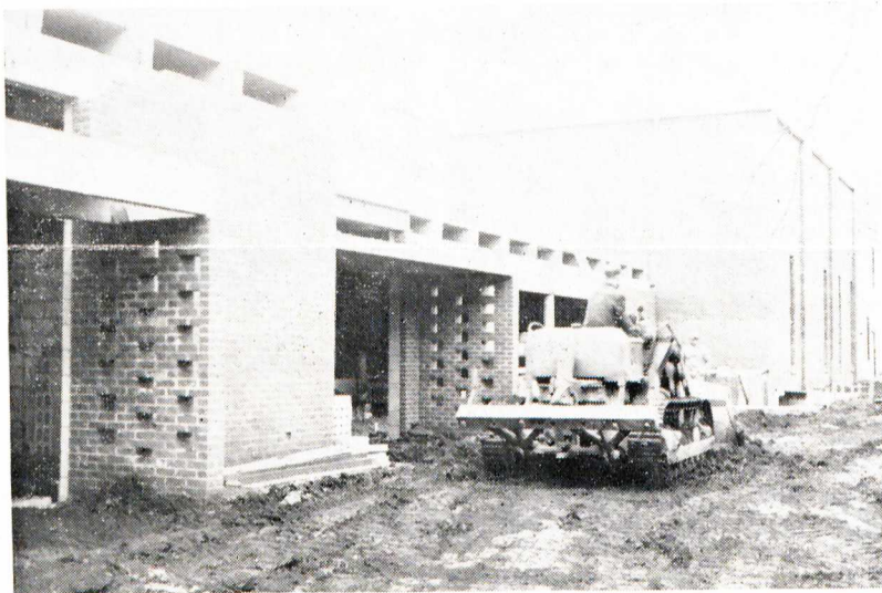
The final phase of excavation and grading is being completed as the bulldozer operator smooths the entrance way to the south side of the new Dining Hall and Student Center. Beyond the bulldozer can be seen the addition to the auditorium. Under this section is a basement approximately 30 x 40 feet which will accommodate a large storage room, heating plant, and rest rooms.
