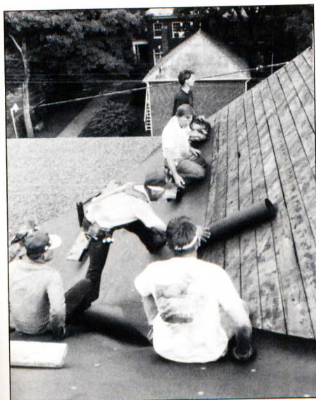
Tarpaper is rolled out before they begin to nail on shingles.
