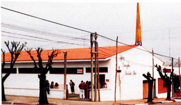
September, 1995, Rivera, Uruguay—WNAC gave over $8000 from the Eunice Edwards Loan Fund for Churches Abroad to help in the renovation of the church building. Mary R. Wischart attended the dedication service.
