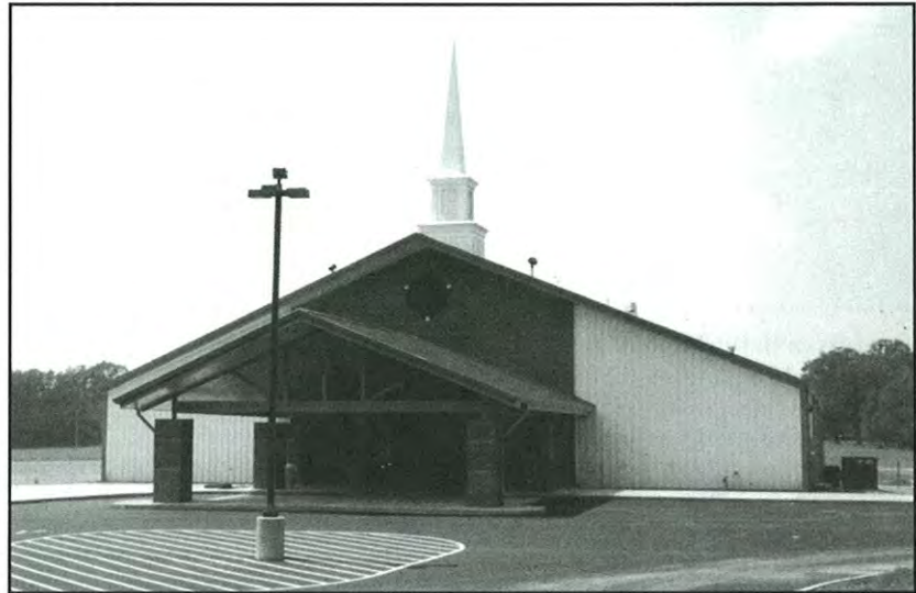
New building at First FWB Church in Jonesboro, AR.
