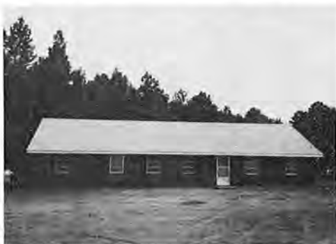
Pictured above is the newly constructed Fellowship Free Will Baptist Church near Micro, North Carolina.
