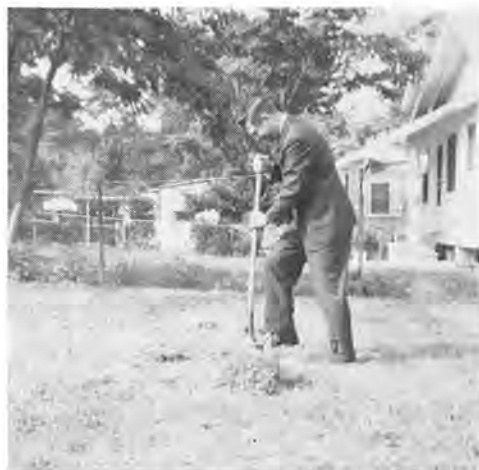
Home Missionary Ken Walker turns spade of dirt during ground-breaking service for new $50,000 church to be built in Washington, D. C. Completion date calls for congregation to be in building for Christmas service.
