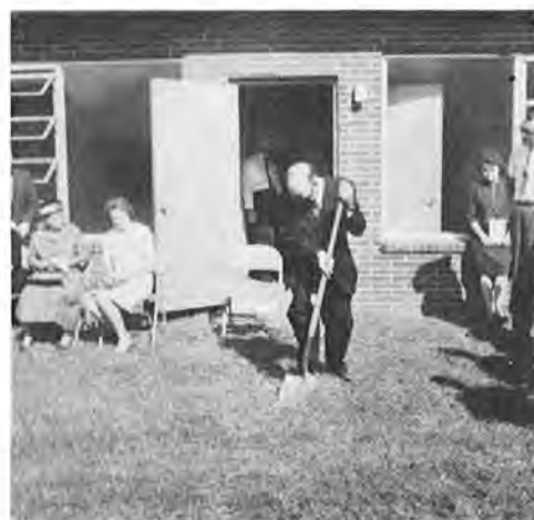
Damon C. Dodd, Pastor of Horton Heights Church, Nashville, Tennessee, turns spade of dirt in ground-breaking exercises for a chapel seating approximately 250. Estimated cost is $30,000.
