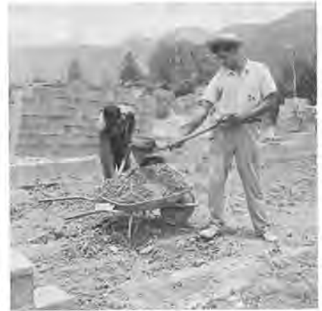
Two of the students prepare the ground for a concrete floor to be poured. This building will be the dining hall and kitchen.
