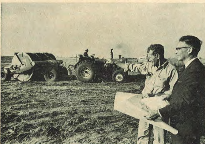
Dr. J. D. O'Donnell is seen looking over the new campus of Oklahoma Bible College in Norman. Four new buildings are now under construction on the 37 acre site. The new facilities will be complete and ready for classes in the fall of 1966.
