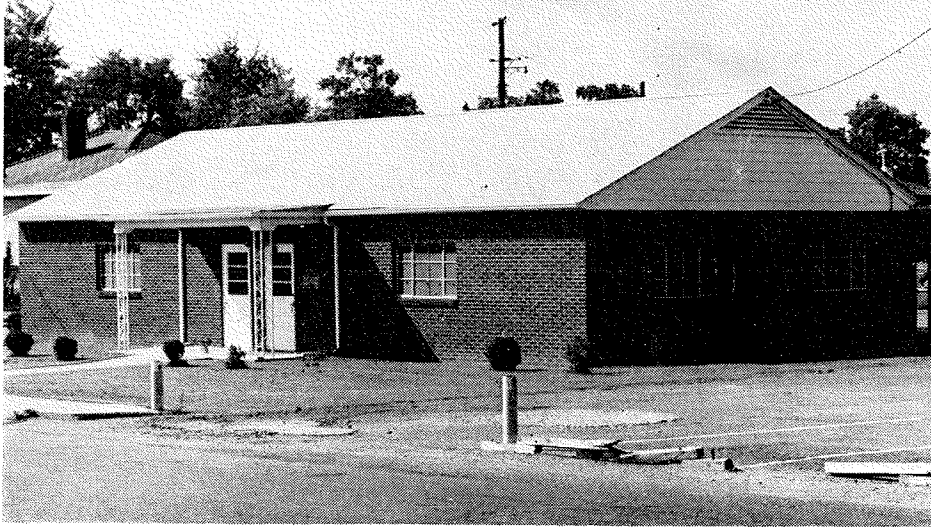
Assembly room was built before classrooms were added.
