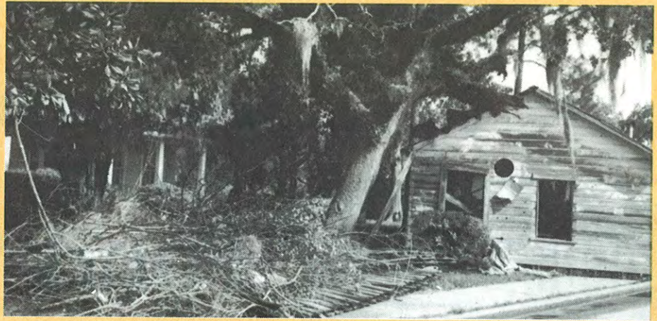
After the flood, the devastation was evident.
