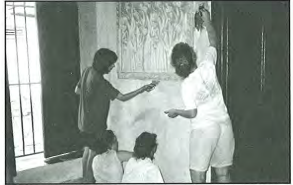
TEAM members help restore the house recently acquired for the FWB Retirement Home.
