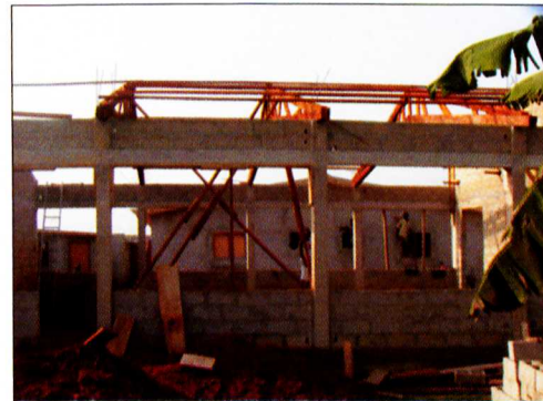
This shot was taken looking through the church to the side of the parsonage...the open spaces in the church will be filled-with decorative blocks-giving light/air.
