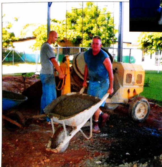
Pouring concrete for addition to building
