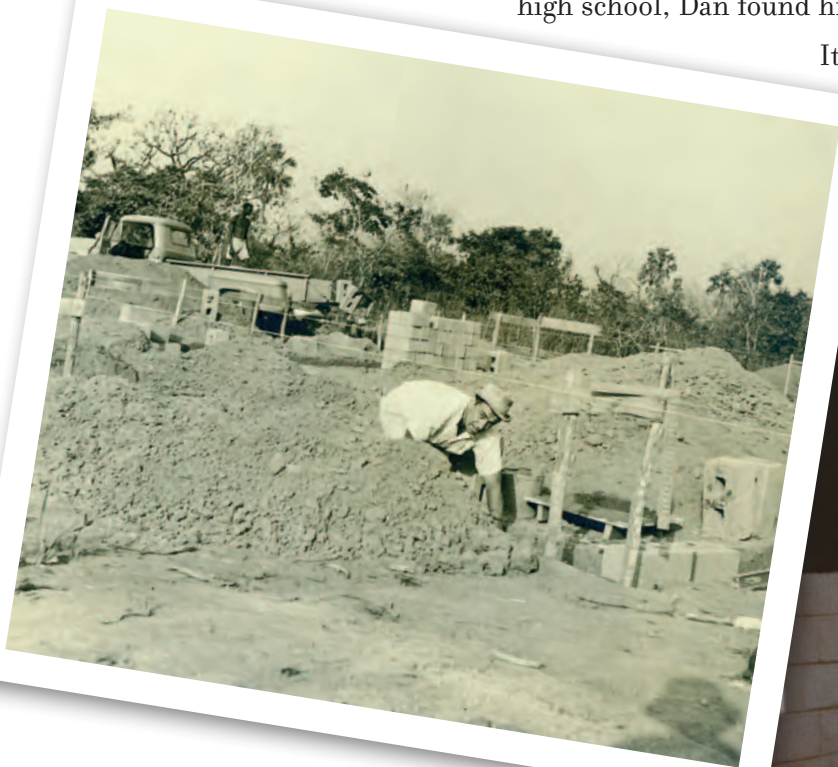
ABOVE: Dan Merkh lays the footing for the foundation of the Doropo clinic.
