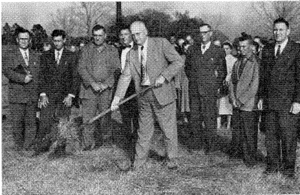
The first step toward construction of a sanctuary for the new church at Chipley, Florida, was the ground-breaking ceremonies conducted January 17. Watching Mr. M. M. Owens turn the first shovelful of dirt are (left to right) Rev. Rufus Hyman, first pastor of the church; Henry Hayes, Joe Revis, Ernest Owen, Cauley Owens and W. B. Usery, building committee, and Rev. W. B. Hughes, present pastor.
