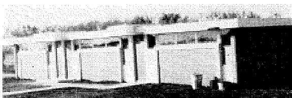
Dormitory for Men
