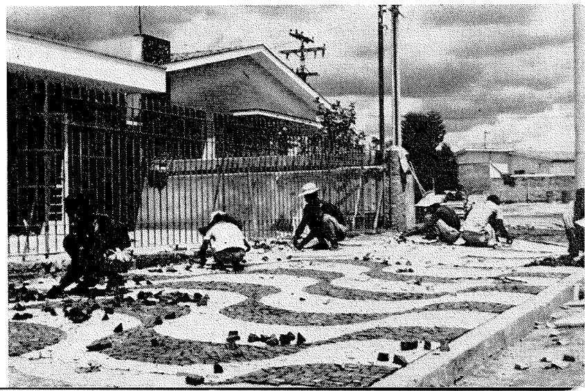
Brazilian worker in Campinas is pounding rock into the ground for construction of a sidewalk.
