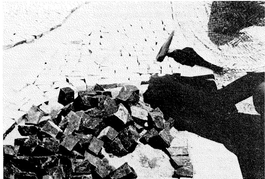
Brazilian worker in Campinas is pounding rock into the ground for construction of a sidewalk.
