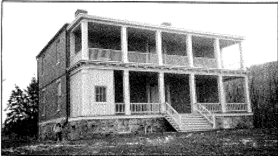
The Lockwood House was considered the main building since it was one of the original buildings donated to the college. Storer College Alumni have restored this building, both inside and out. It contains a completely restored schoolroom similar to the period of the post Civil War. (Kelley and Ashley Joslin at left of building.) The house is usually open to the public.
